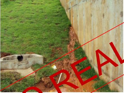
MECHANISM - 2 THROUGH CUTOFF TRENCH AND FOUNDATION
