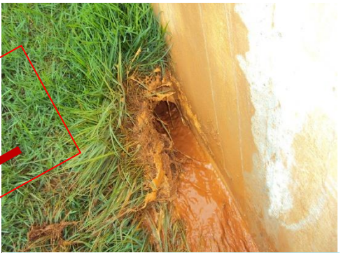
MECHANISM - 2 THROUGH CUTOFF TRENCH AND FOUNDATION
